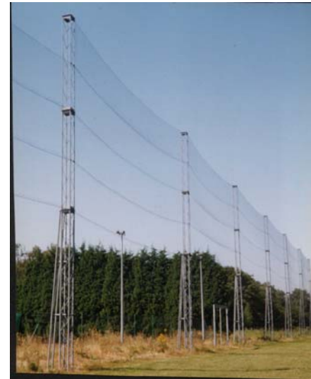
Towers and Netting Used to a height of 15m
