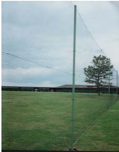
Framework and Netting Used to a height of 6m
